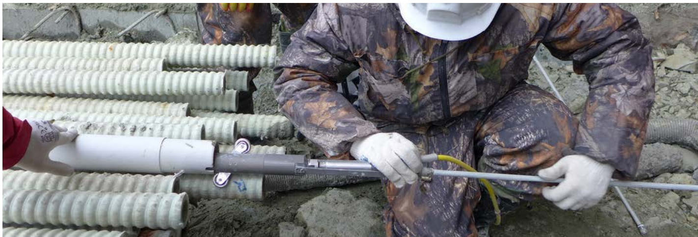
Preparing T-REX probe for horizontal surveying
